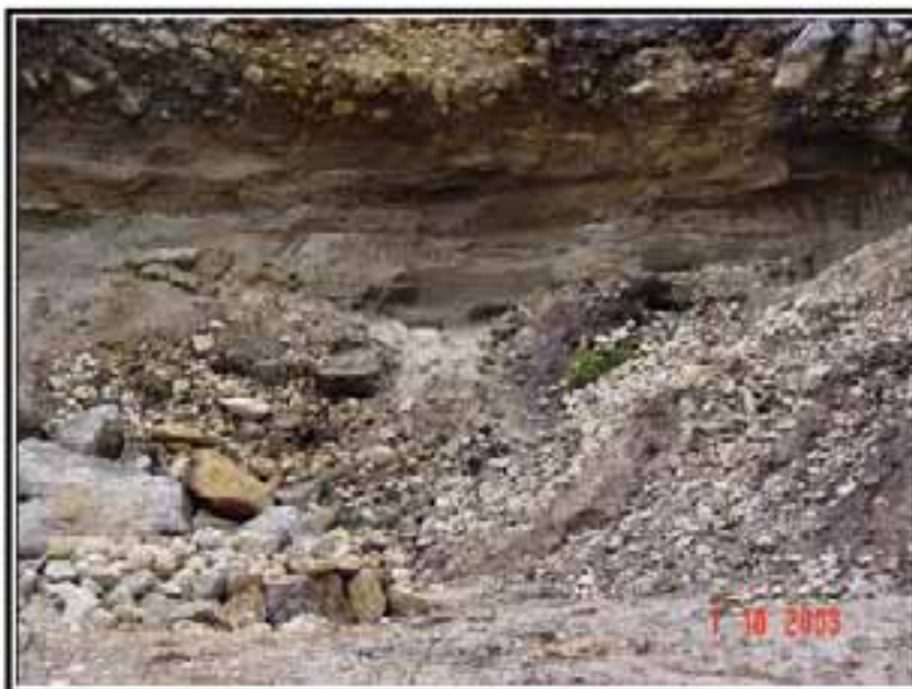
Plate 2.22 Collapse of old depositional landforms due to road building downstream of Thangu
