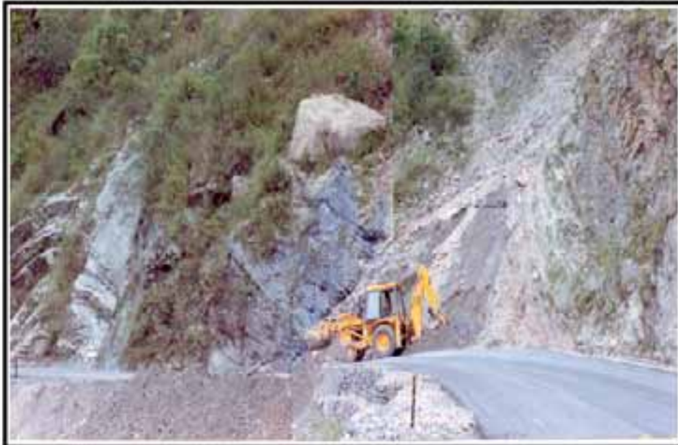
Plate 2.16 Berrick landslide showing a fault propagated fold and the circular failure of carbonaceous phyllite
