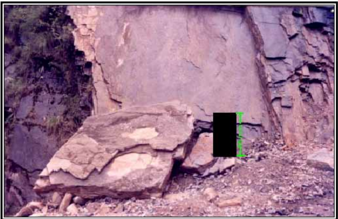
Plate 1.4 Rhombohedral blocks separated out from the rock mass by plane failure mode
