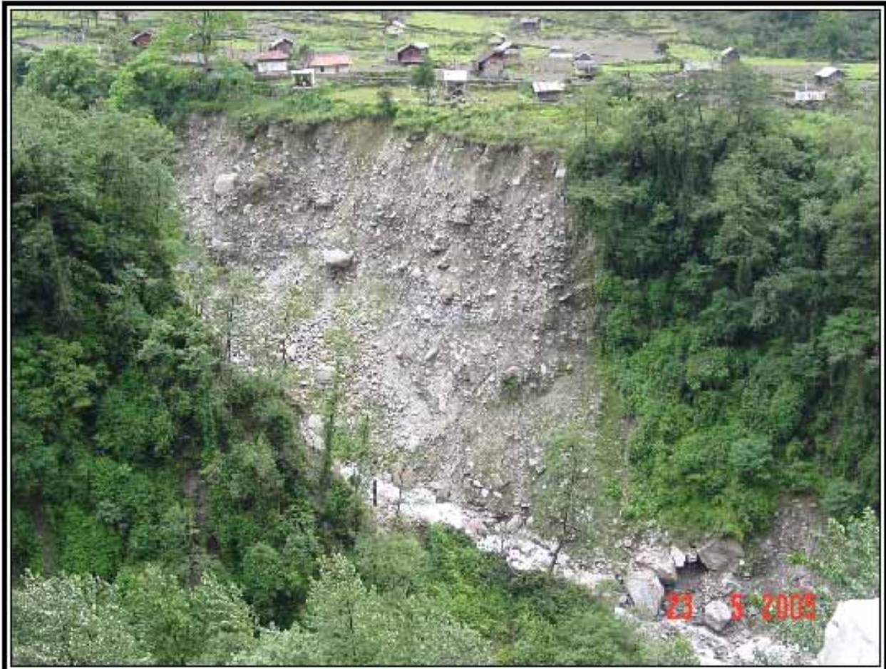
Plate 1.10 Collapse of Terrace on the left bank of Lachung and Creeping of settlement on it
