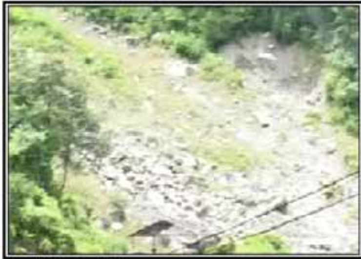
Plate 2.7 Lanta Khola Landslide
